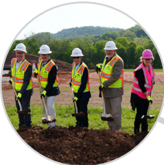
Messer Expands in Berryville with New Air Separation Unit.
